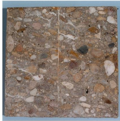
Concrete reinforced with FIBRAFLEX fibres Aspect after 15 months
